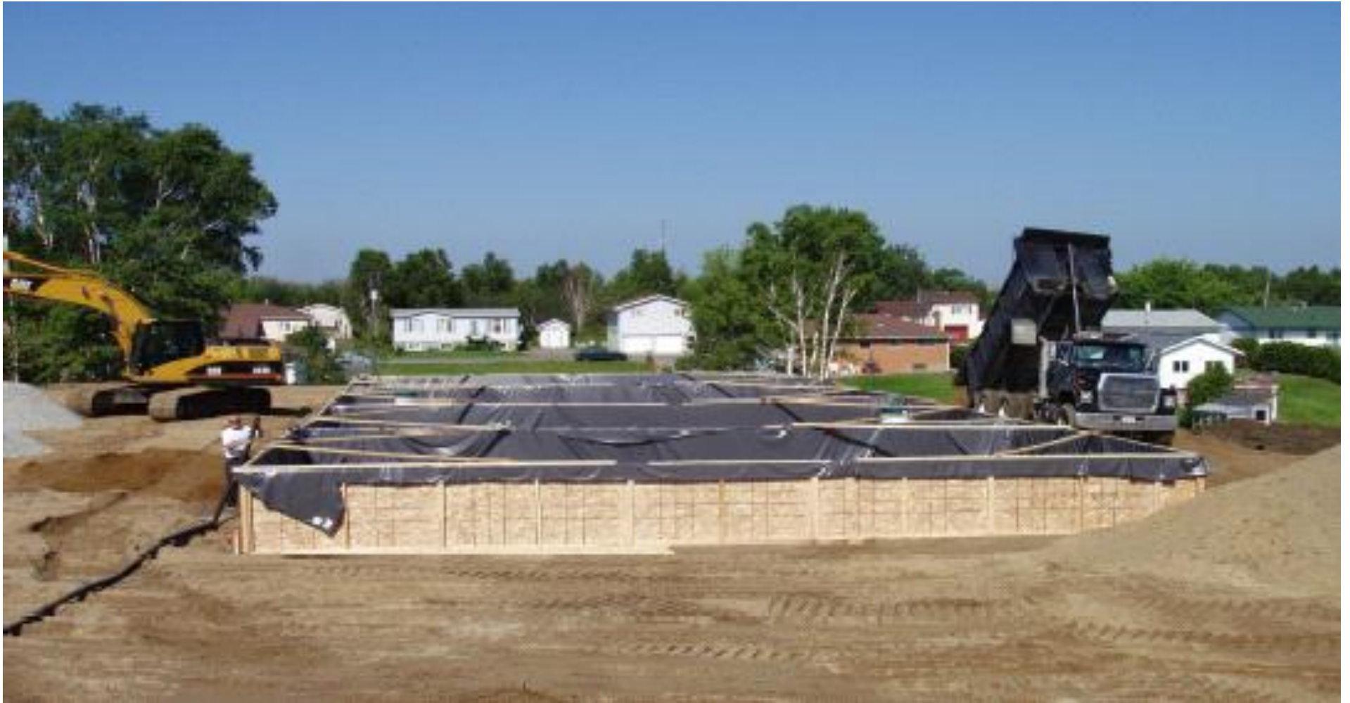
Valley View Public School, Sudbury. Liner and plywood forms. Aqua Wetland System www.aqua-tt.com
