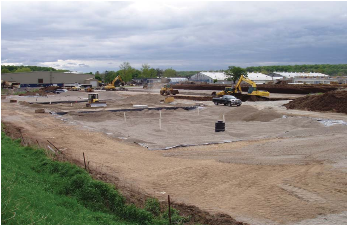
Figure 11 Installation of 28" either industry standard concrete sand, 1/4" gravel or a mixture of concrete sand and pine wood shavings, depending on treatment objectives etc.
