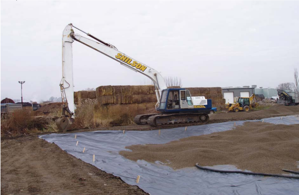
Figure 10 Installation of 1/2" clear stone over top of Big 'O' collection piping. The media on top of this gravel layer consists of 28" of either industry standard concrete sand, 1/4" gravel or a mixture of concrete sand and pine wood shavings, depending on treatment objectives etc.
