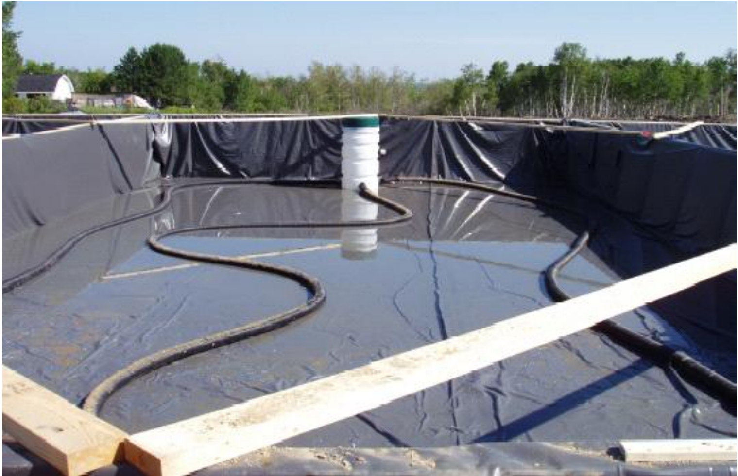
Drainage piping.
