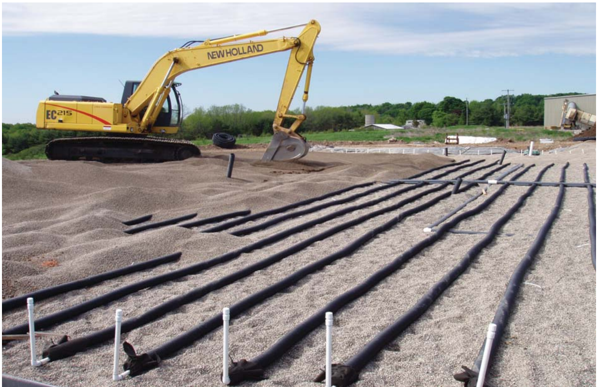
Figure 13 Installation of 'Winter' dosing manifolds. Manifolds are covered with 6-8" of 1/2" clear stone. This clear stone is then covered with a final layer of sand. Peat moss may be mixed with this sand using a 50:50 ratio.
