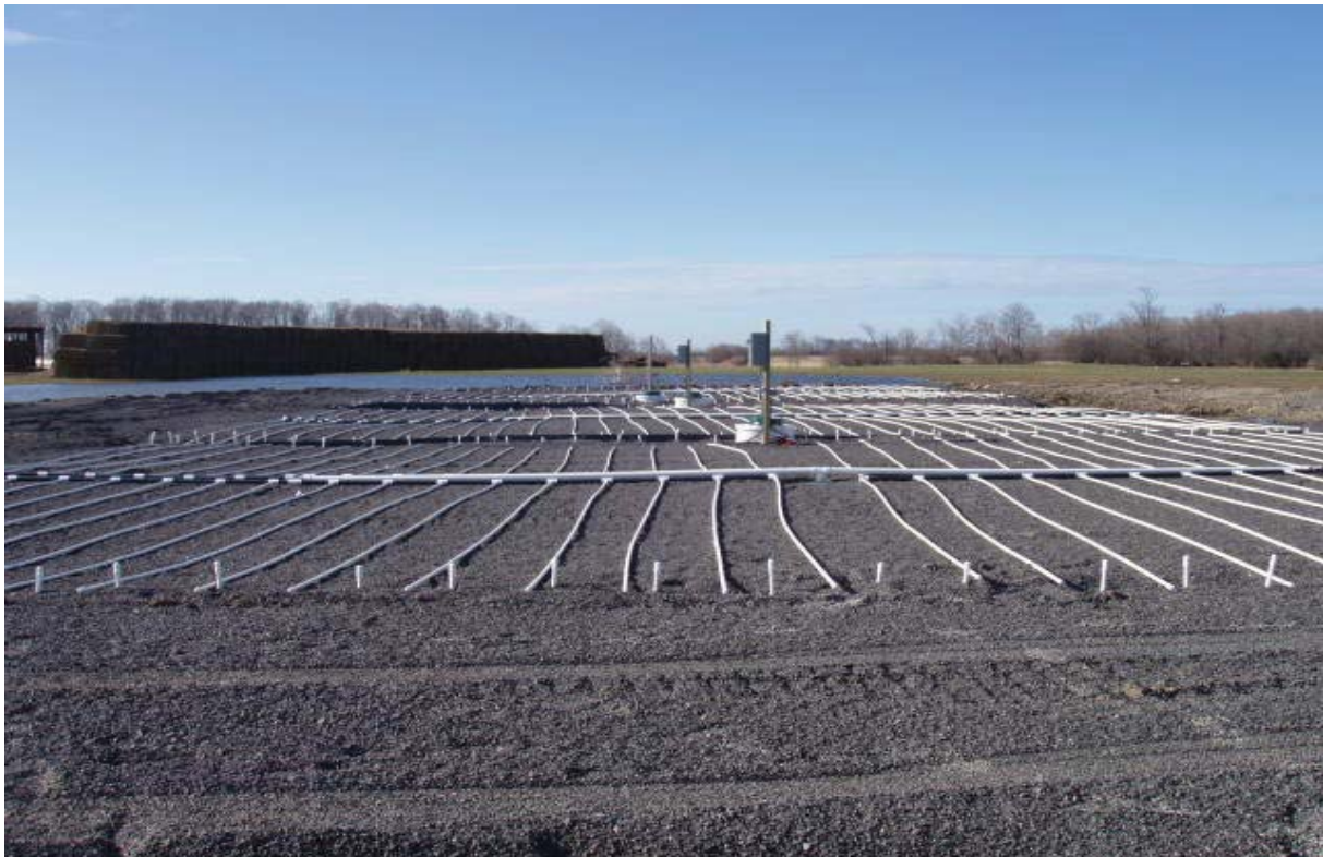
Figure 15 View of 'Summer' dosing manifolds. These manifolds are located on top of the cell surface. These manifolds are located directly on top of the final layer of sand. Peat moss may be mixed with this sand using a 50:50 ratio.
