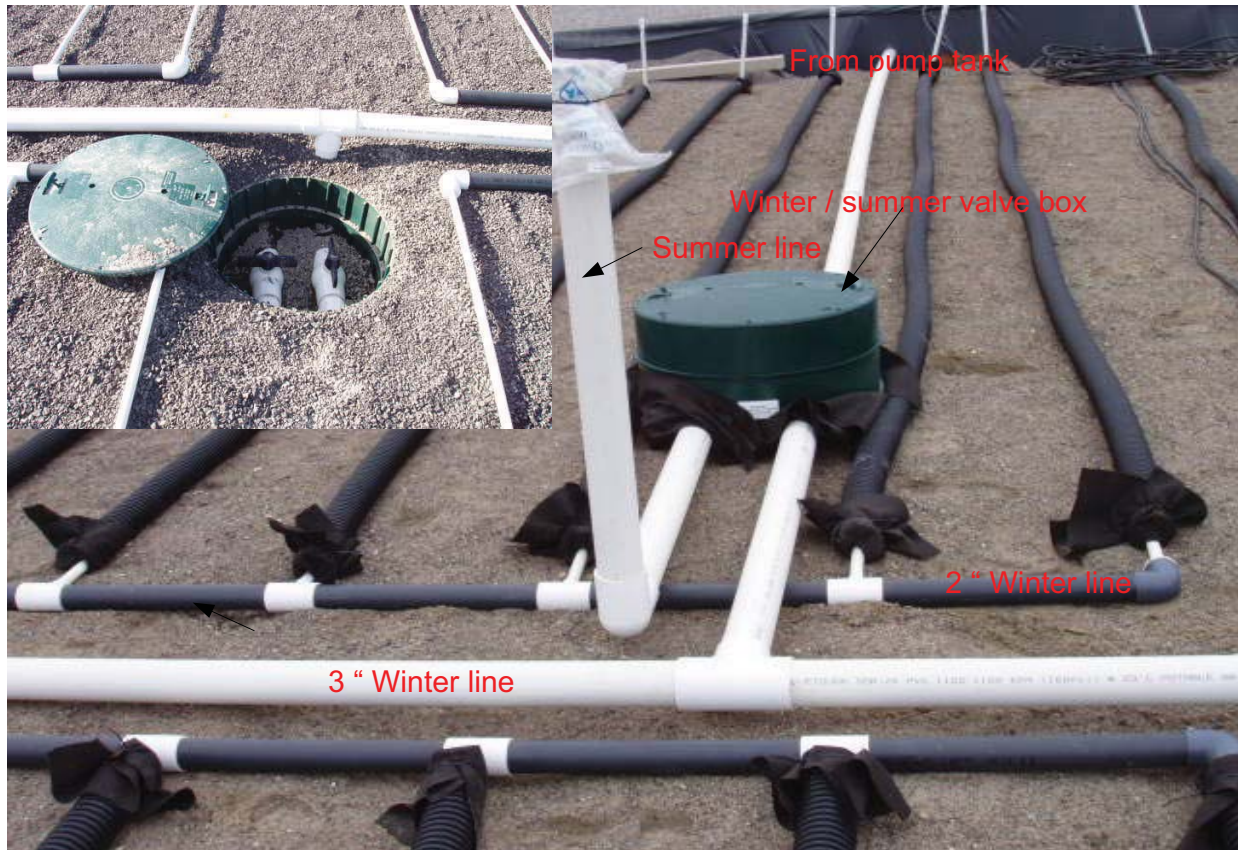
Figure 14 Additional manifold detail.
