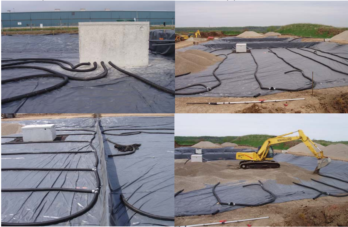
Figure 8 Installation of pump tanks. Tanks can be either concrete or plastic depending on availability and size etc. Perforated Big 'O' collection piping allows the water from the bottom of the cell to drain into the pump tank. Big 'O' pipe is covered by 12" of 1/2" clear stone to prevent infiltration of sand media into collection pipe.
