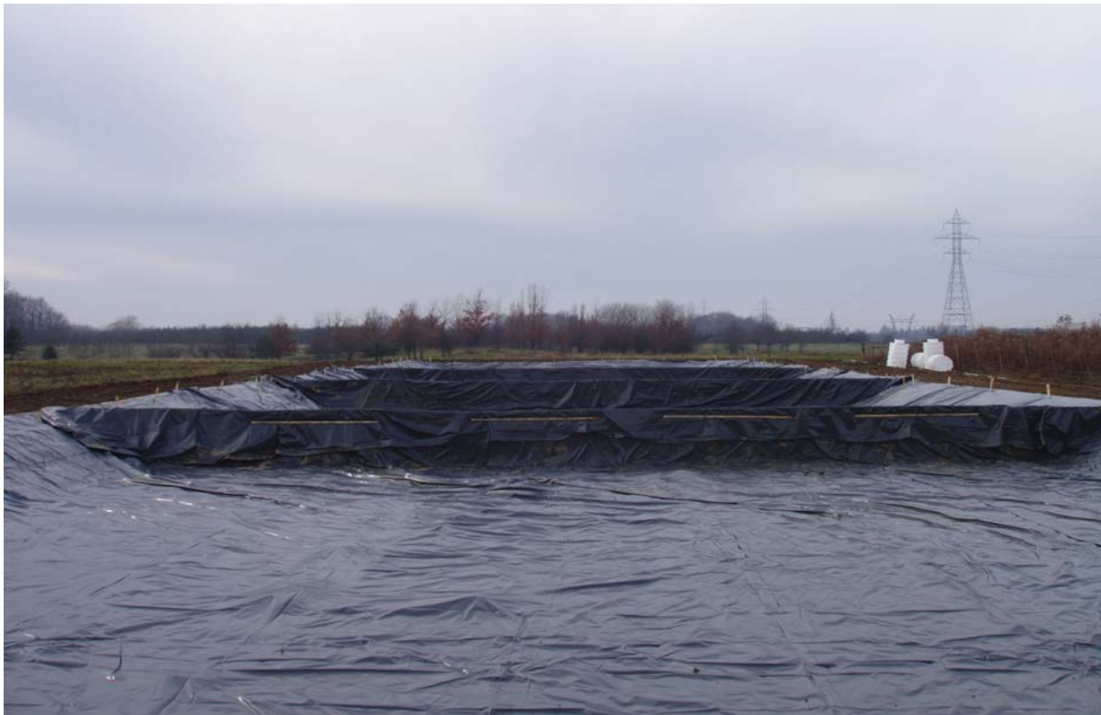
Figure 7 Liner installation complete.
