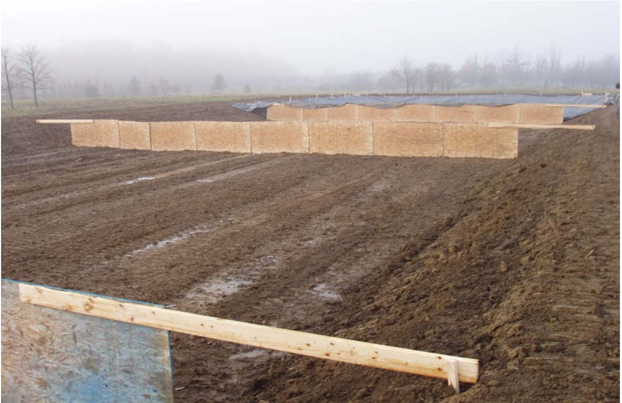
Figure 4 Cell wall construction continued. Wall slopes are accommodated using 2X6 spruce timbers from top of plywood to top of berm.
