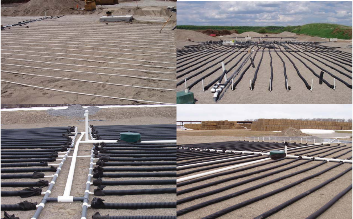
Figure 12 Installation of 'Winter' dosing manifolds. These manifolds consist of 3/4" PVC pipe with 1/4 holes drilled ~4' on center. The 3/4" pipe is encased with 3" diameter perforated Big 'O' pipe with 1/2" holes drilled 2' O/C. The 3/4" pipe is connected to 2" schedule 40 PVC headers which in turn are connected to 3" Schedule 40 PVC dosing lines. Winter dosing manifolds are covered with 1/2" clear stone (Figure 13).
