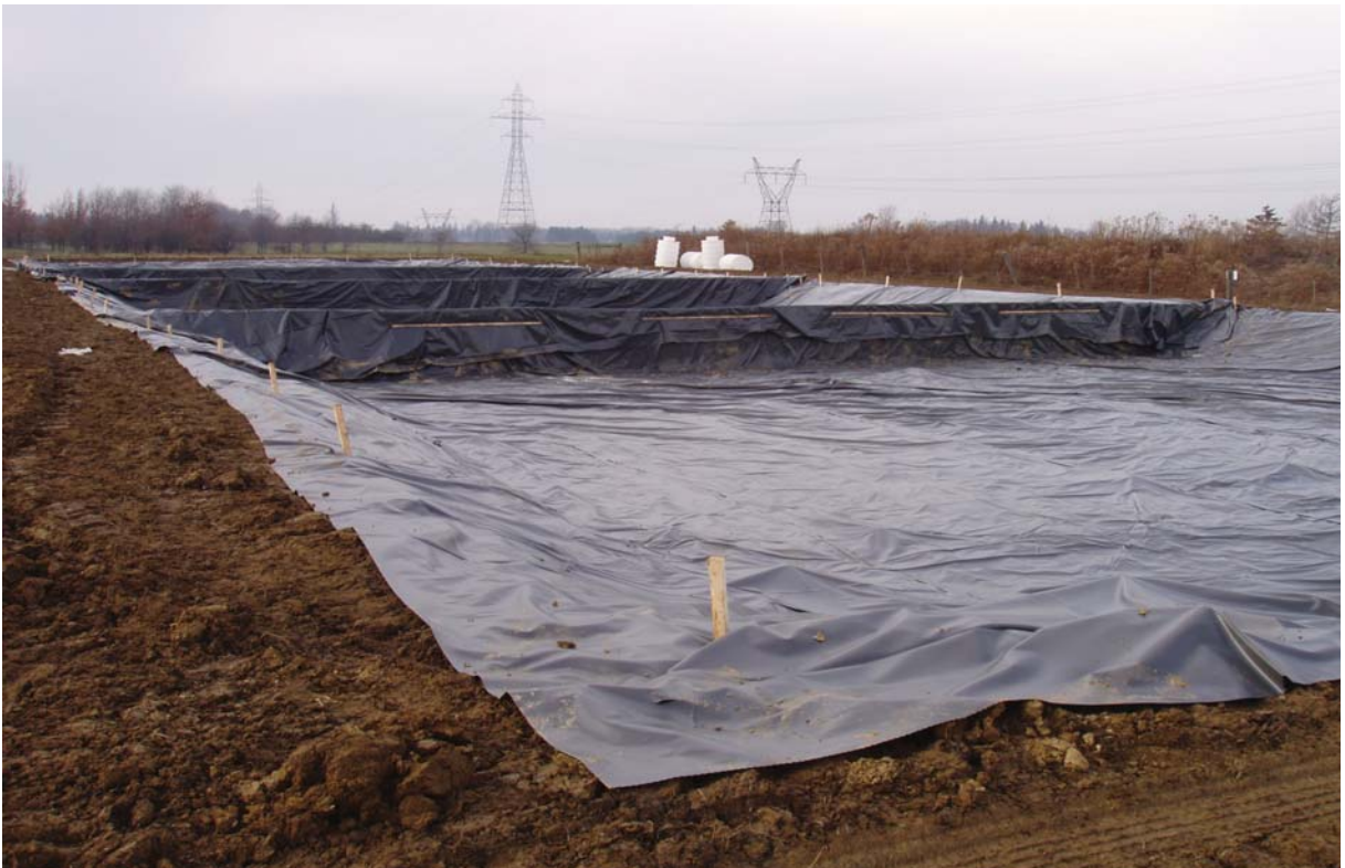
Figure 5 Installation of PVC liner. The liner edges are secured along the berm via wooden stakes. The liner is draped over the cell walls (Figure 6).
