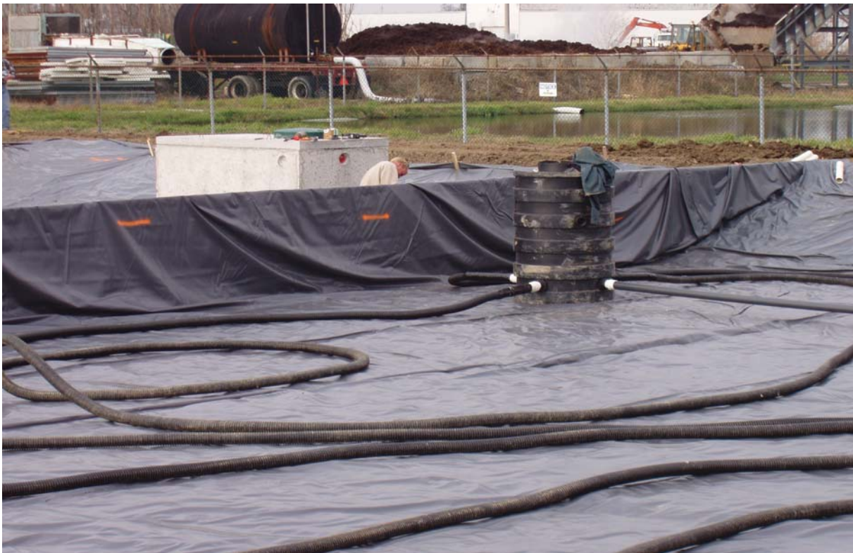
Figure 9 Poly pump barrels can be used in place of concrete tanks. These are easier to install and handle.
