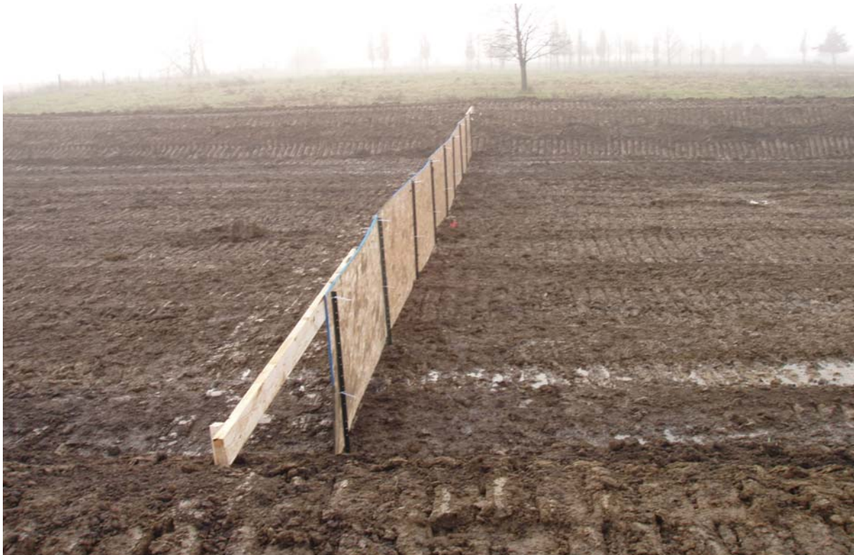
Figure 3 Cell walls are built using plywood. Plywood panels are secured to iron T-bars driven into the earth. Wall slopes are accommodated using 2X6 spruce timbers from top of plywood to top of berm (figure 3).
